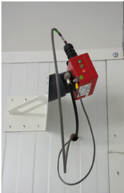
The powder-coating booth is fitted with a fire-suppression system. In the event of spark generation, the monitoring system triggers the extinction with CO 2 and other measures.
