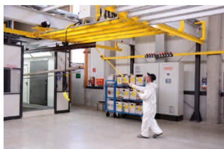
The lifting beams are pushed manually to the traversing gantry; the transport in the traversing gantry is handled electrically.
